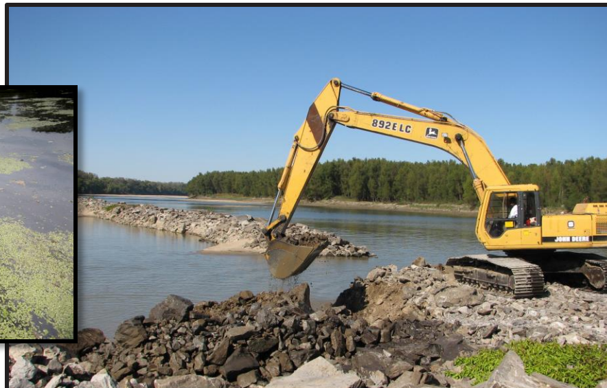
Dike notching connects secondary channels and isolated wetland areas to improve habitat.
